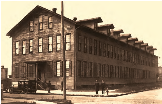
The Ybor Oliva project will add tall, narrow windows and new siding to restore historic character to the former cigar factory (shown above). Photo courtesy of Oliva Tobacco Company and A-Investments Development Corp.
